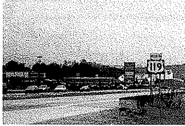
TERRADON's design for the 4 to 6 lane widening of US 119 in Kanawha County won the WVDOH's Engineering Excellence Award for 2000. The design was completed in June of 2000.
