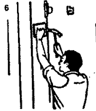
Is the panel plumb?
