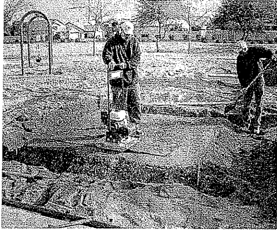
Start with a base of compacted aggregate
