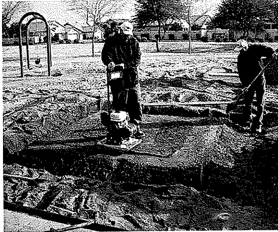
Start with a base of compacted aggregate
