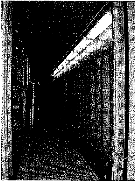
Interior view of reverse-osmosis self-contained, modular treatment unit
