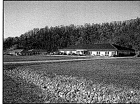
The home office of Thrasher Engineering is located in Clarksburg, WV
