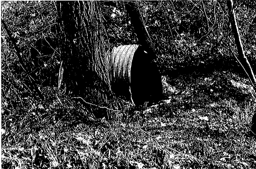
Figure 1D—Mine drainage at railroad cross drain outlet
