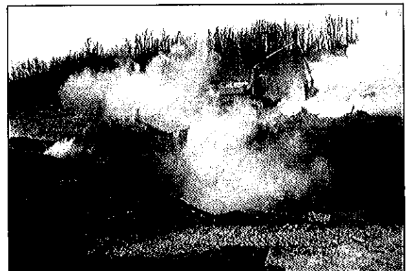
Jamison Burning Refuse Reclamation Project
