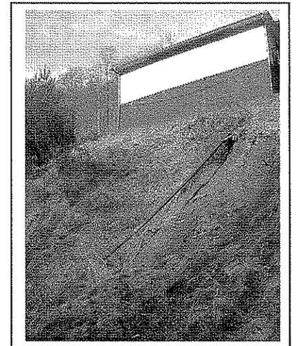
Above Picture: This shows the slide under cutting the foundation of the residential structure. The toe of the slide was severely saturated with mine water which greatly increased the likelihood of further movement.
