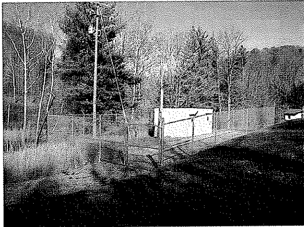
50 GPM Wilsontown Booster Station
