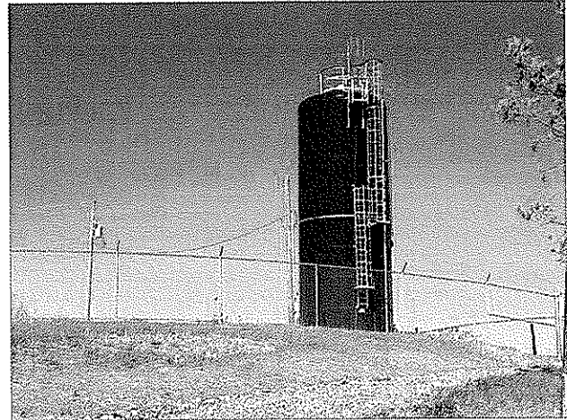
43,000 Gallon Salem Ridge Water Storage Tank
