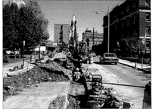
Completed in 2003 Main Street Waterline Replacement Project New 12" Ductile Iron Pipe Installation
