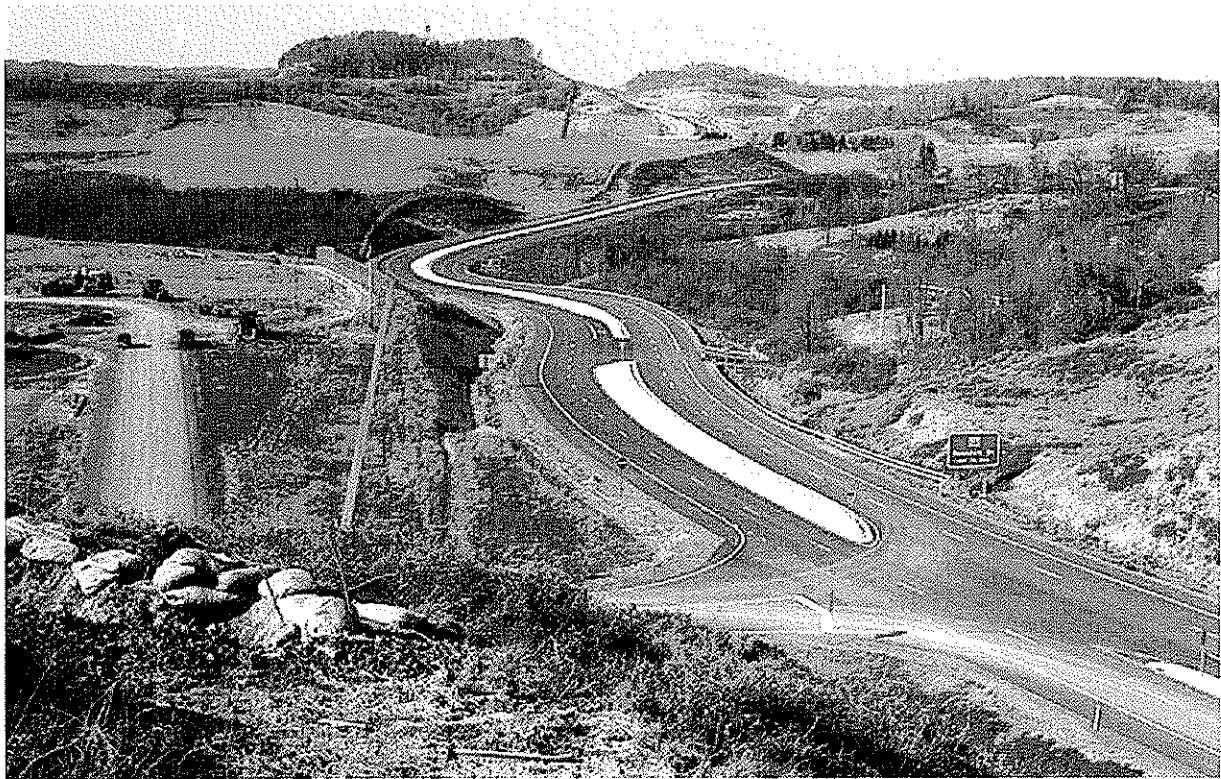
ROUTE 279, NORTH BRIDGEPORT BYPASS - COMPLETED IN 2000
