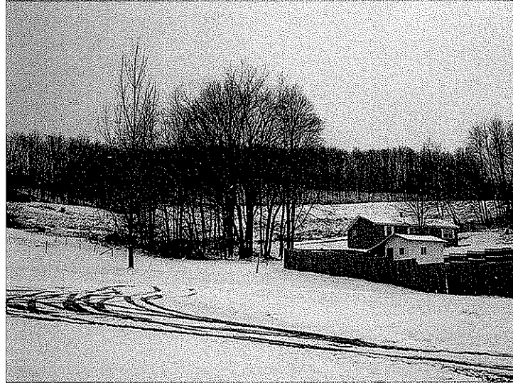
Figure 1—View facing south from Locust Avenue toward the project site, including mine portals
