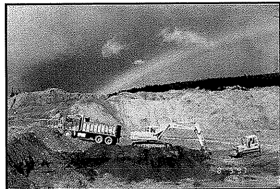
Removal of tailing from floodplain
