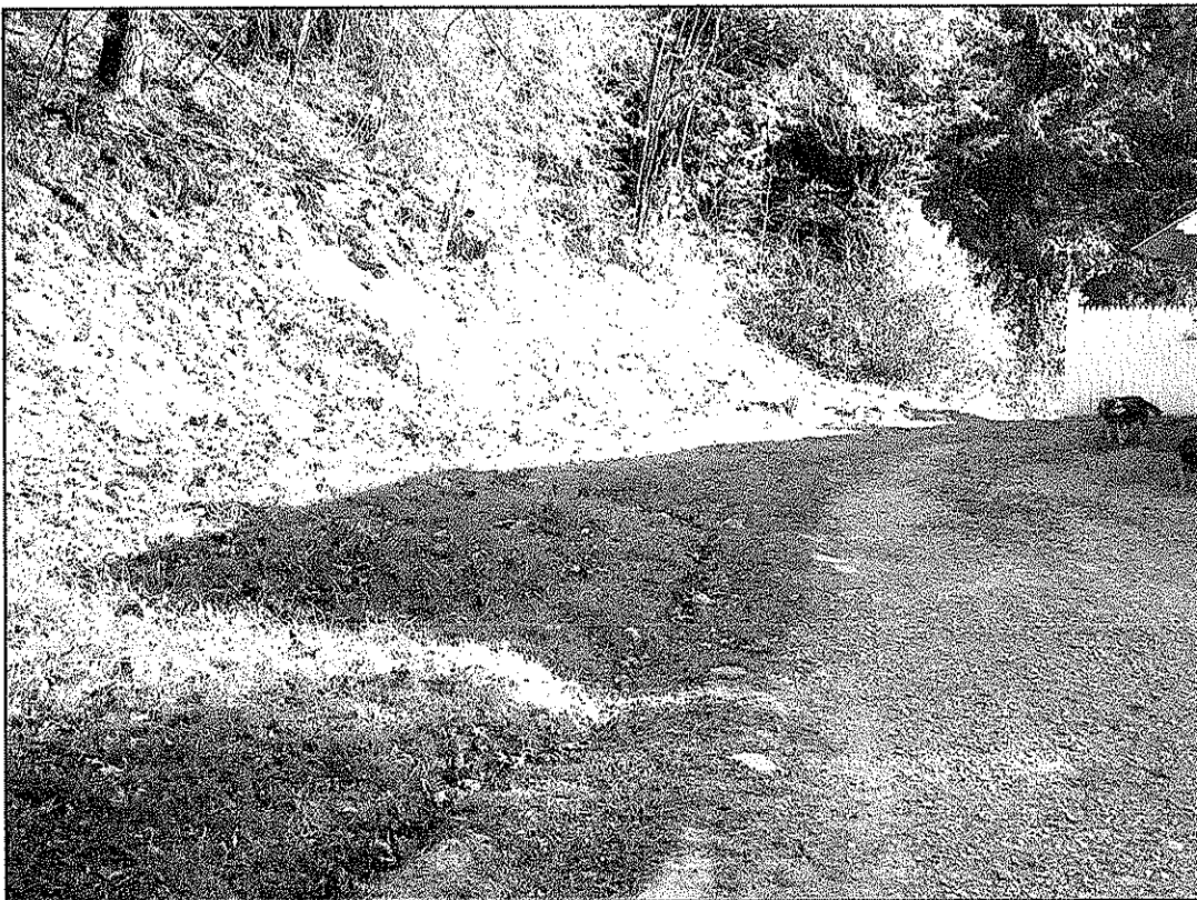
Matoaka (Young) – DITCH ALONG REAR OF DRIVEWAY TO COLLECT SEEPAGE
