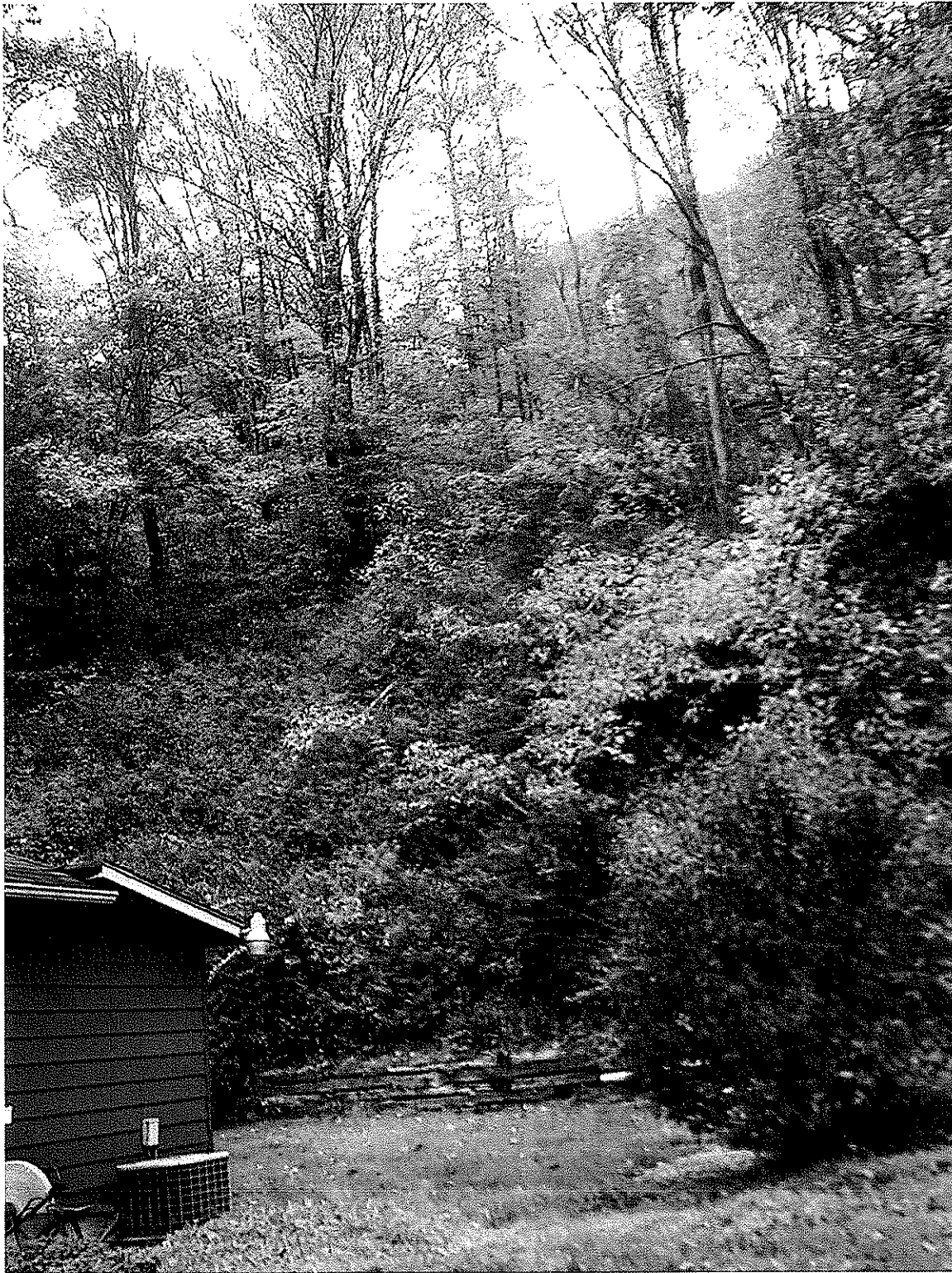
Figure 2—Landslide Behind Mr. Oakley's House
