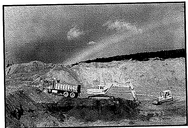
Removal of tailing from floodplain
