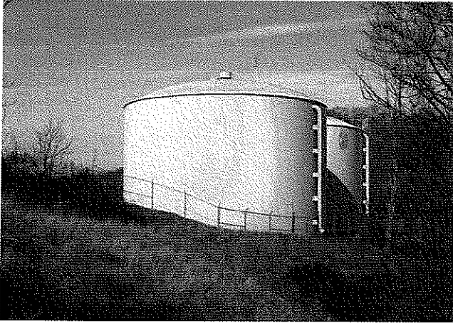
Total Project Cost = $4,400,000; Completed 1994 Two 1,000,000 Gallon Storage Tanks Part Of FBI Water Project
