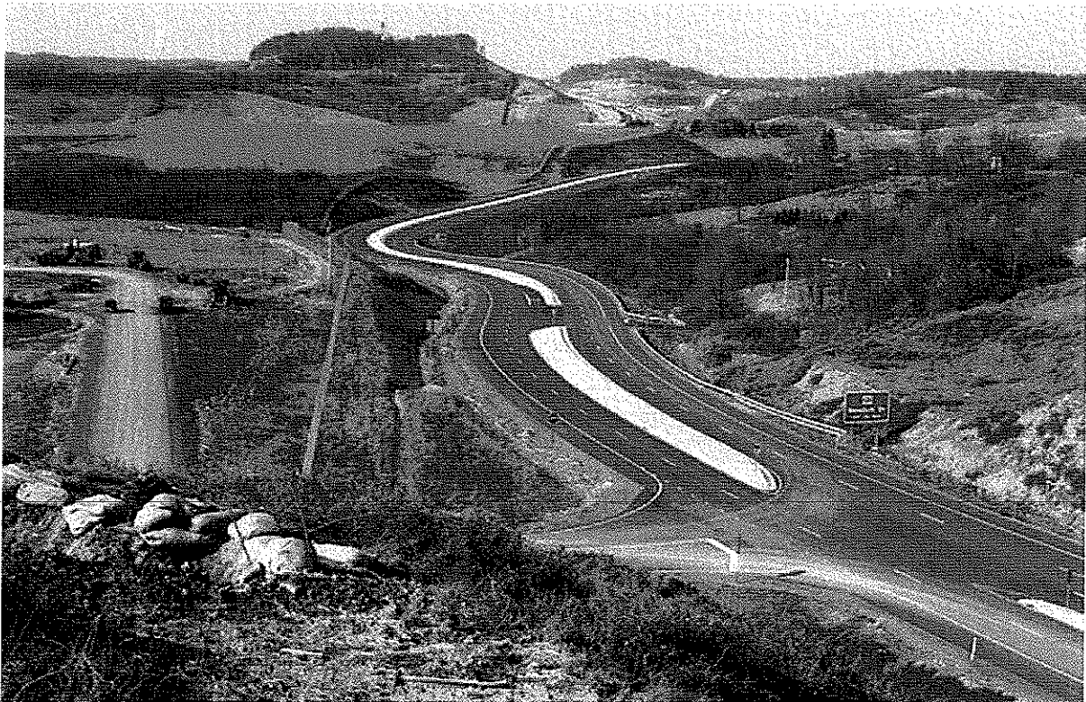
ROUTE 279, NORTH BRIDGEPORT BYPASS - COMPLETED IN 2000
