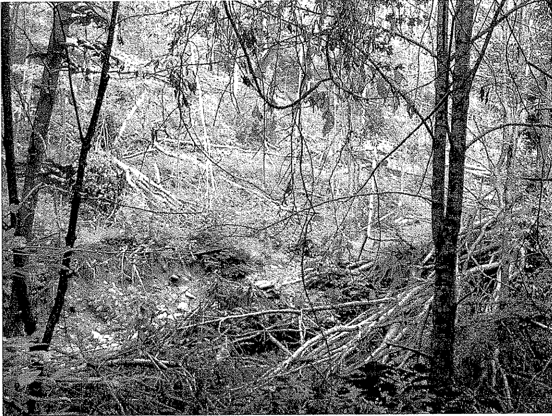
Figure 6--The Slide Area Encroaching on the Stream
