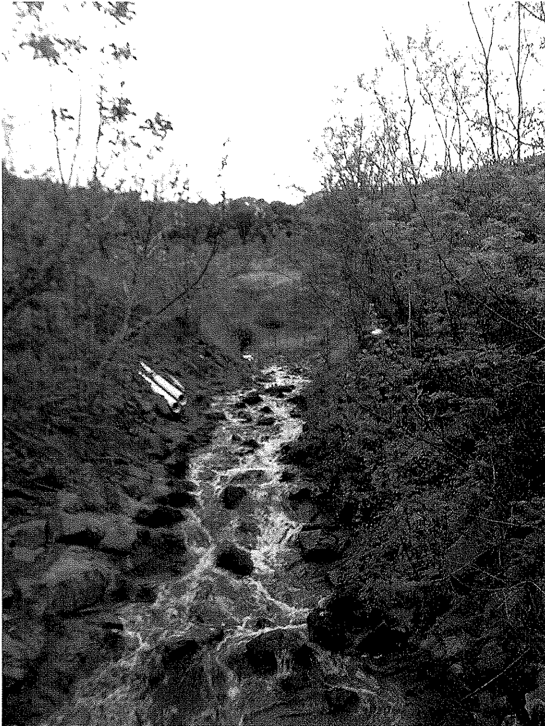
Figure 7—Stabilized Refuse Slopes and Channel with Under Drain Outlet
