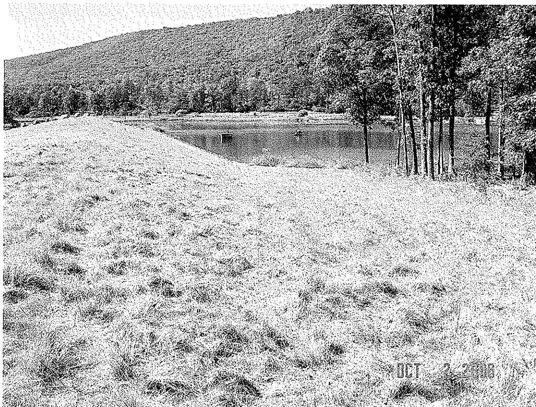
WARDEN LAKE DAM MODIFICATION, HARDY CO., WV
