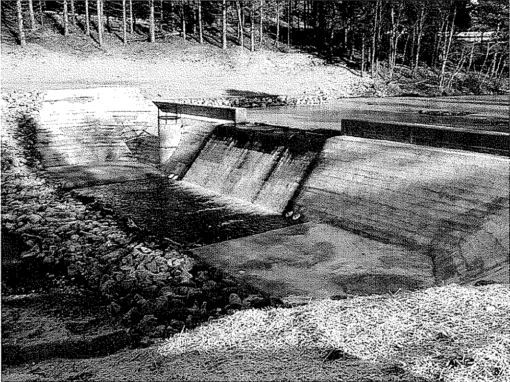
THOMAS DAM MODIFICATION, THOMAS, WV
