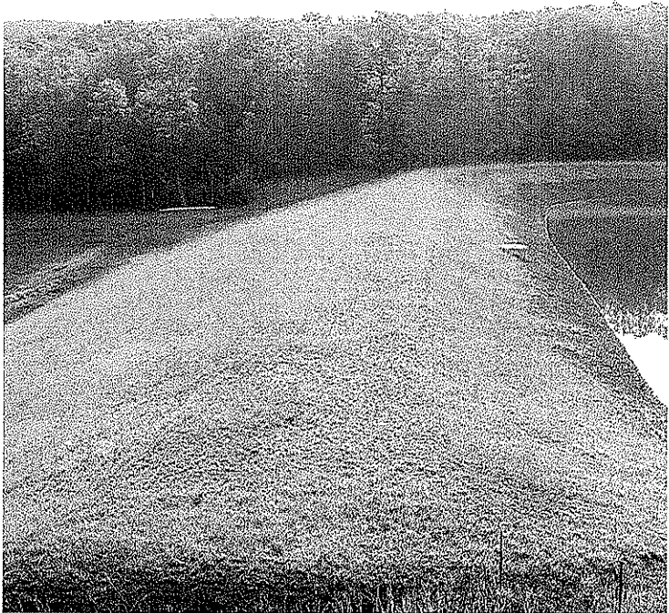
WILSON DAM MODIFICATION, HAMPSHIRE CO., WV
