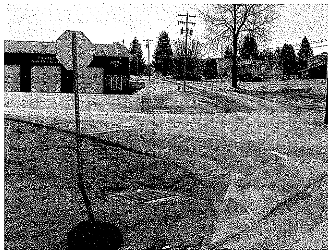
New Storm Drains and Catch Basins
