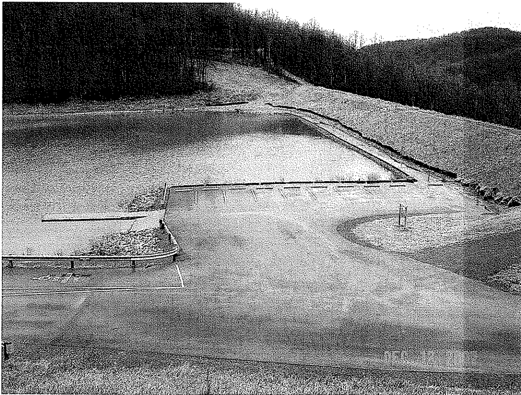
BAILEY DAM MODIFICATION, MONONGALIA CO., WV
