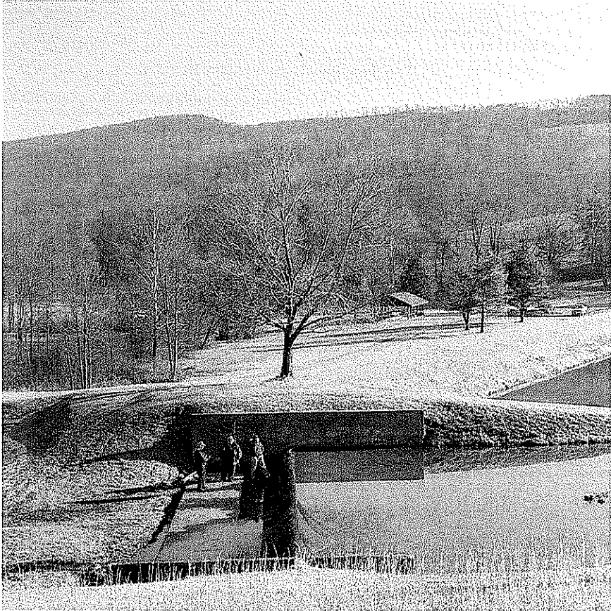
BELINGTON DAM MODIFICATION, BELINGTON, WV
