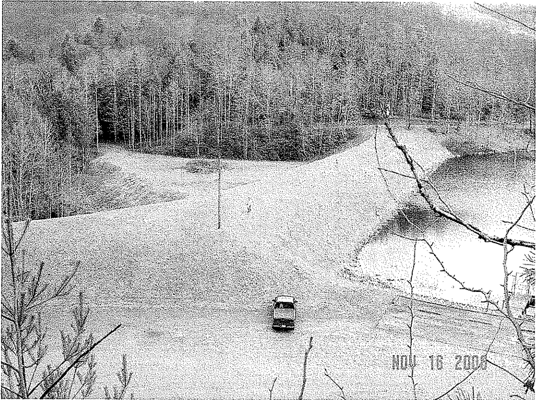
PLUM ORCHARD DAM MODIFICATION, FAYETTE CO., WV
