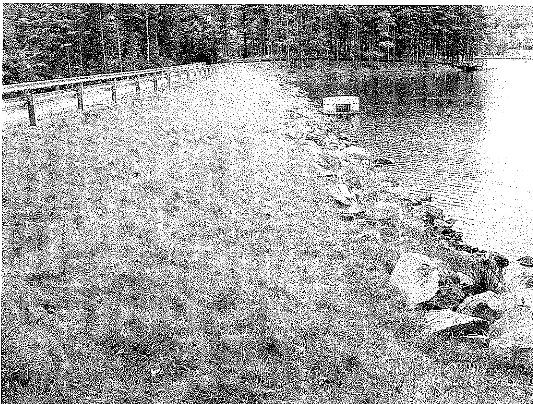
MONCOVE DAM MODIFICATION, MONROE CO., WV
