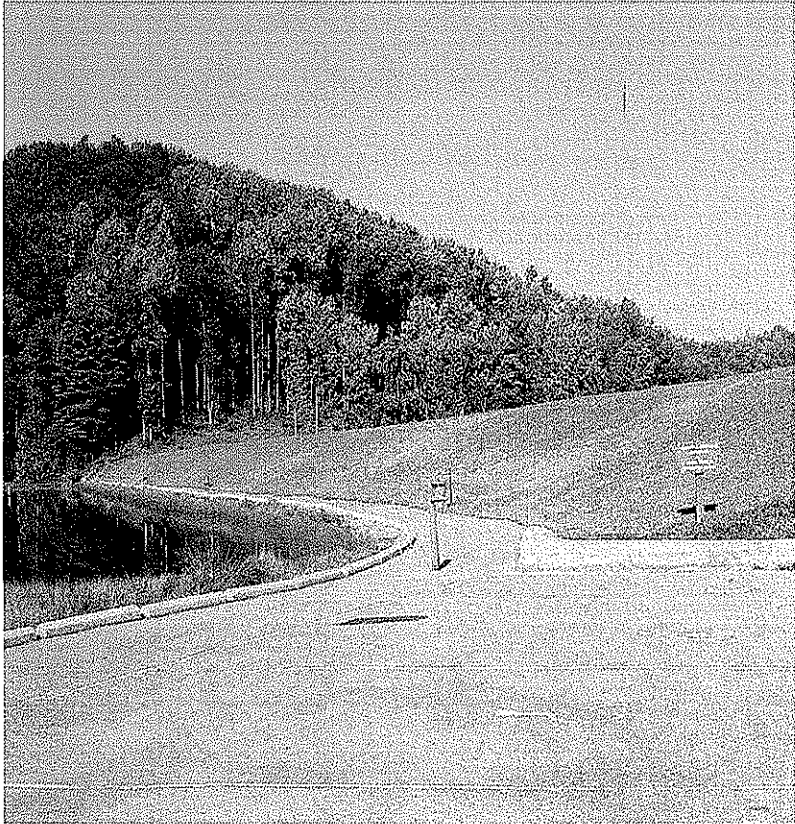
TETER CREEK DAM MODIFICATION, BARBOUR CO., WV
