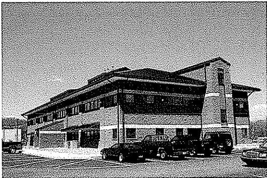
WVDOH District Six Office Building Moundsville, WV
