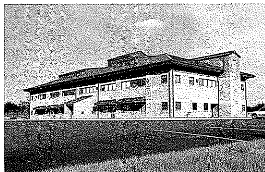
WVDOH D-10 Office Building, Gardner, WV
