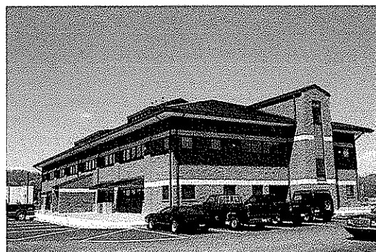
WVDOH D-6 Office Building, Moundsville, WV
