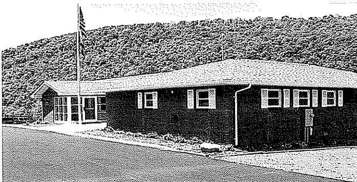
Architectural and Engineering design for new addition and renovations to the detachment in Pendleton. Included in the structure are the following departments: DMV, BCI, 911, & regular squad space.
