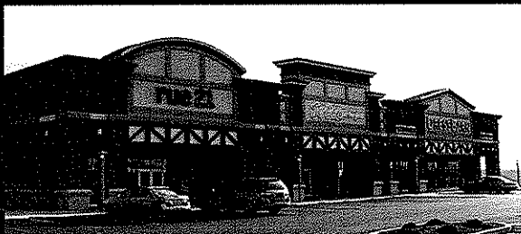
Power Center 'B' Phase 1
