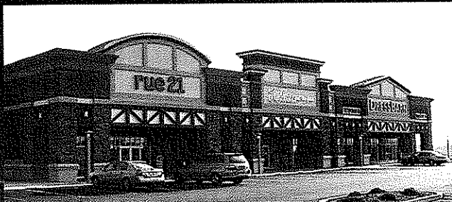
Power Center 'B' Phase 1
