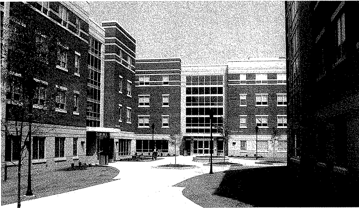
Marshall University Student Housing Complex
