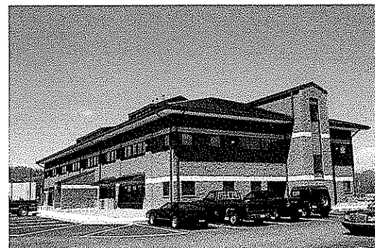
WVDOH D-6 Office Building, Moundsville, WV
