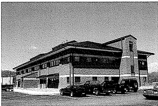
WVDOH District Six Office Building Moundsville, WV
