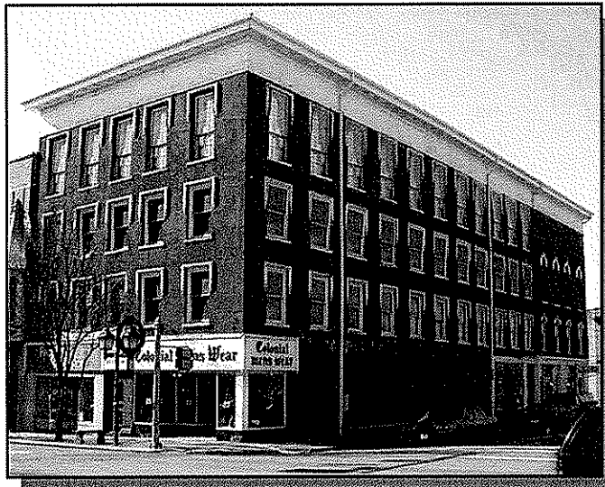
View of northeast corner of the Woodward Opera House
