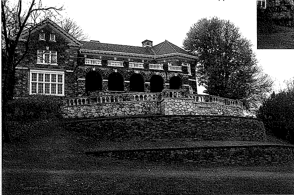
Main Foundation Support Wall
