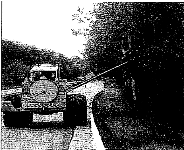
Cutting beyond the guardrail
