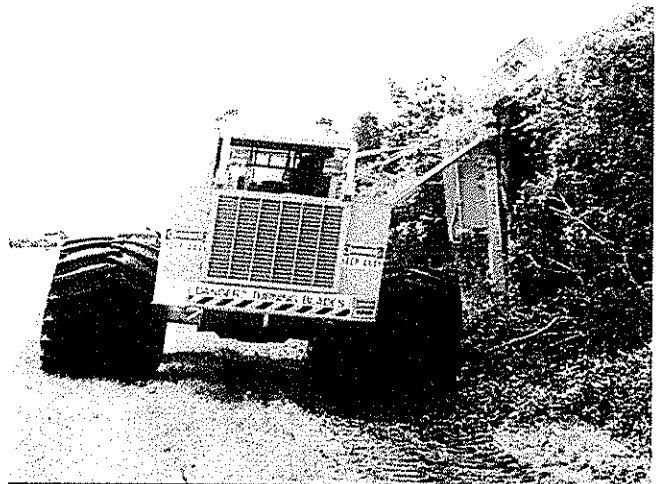
Controlling encroaching brush on right-of-way
