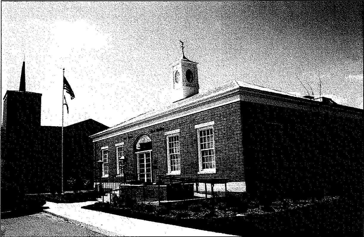
Chapman Technical Group's St. Albans Office
