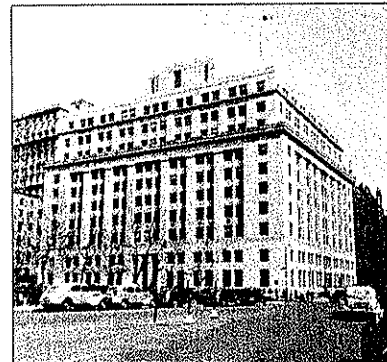
Department of Health Building
