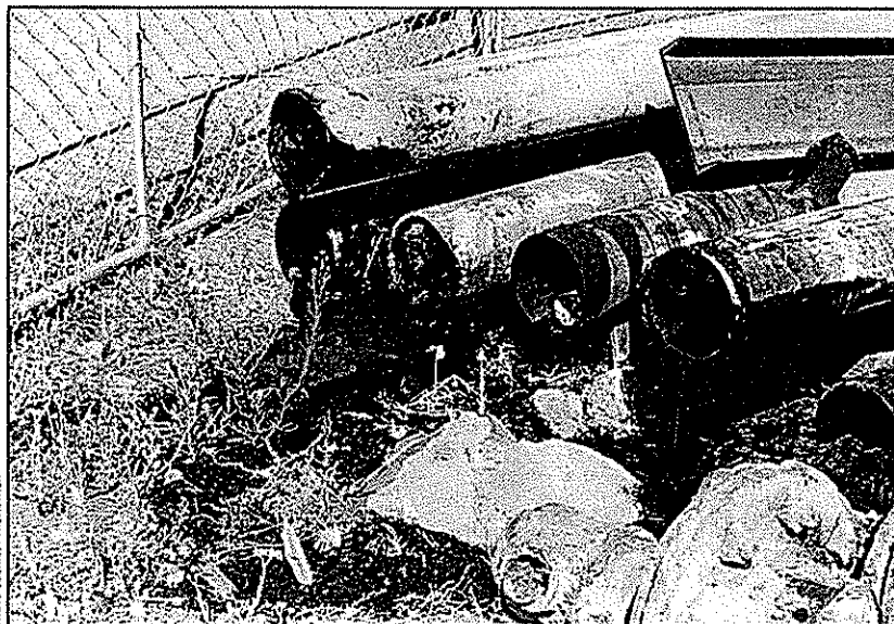
Photo 6. Failure to identify that existing structural steel pipe columns were filled solid with tar required the complete redesign of structural reinforcement during construction.
