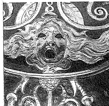
Work on the Medusa started with removal of the original coatings, etching with acid, a coat of epoxy primer, epoxy top coat and applying the gold leaf.
