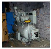
This surplus compressor is used to clean the equipment at the Kanawha County Solid Waste Authority.
