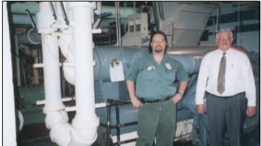
CAMC is sold on the savings at WVSASP. Pictured (l-r) are Dan Brown, Senior Control Technician, and Edwin Rawls, Director of Plant Operations.
