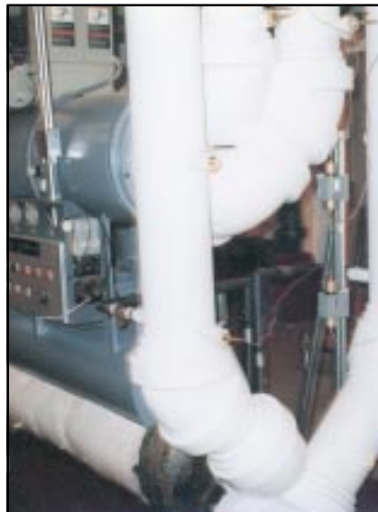
A Closer Look... The surplus chiller unit proved to be a great asset to the Charleston Area Medical Center.
