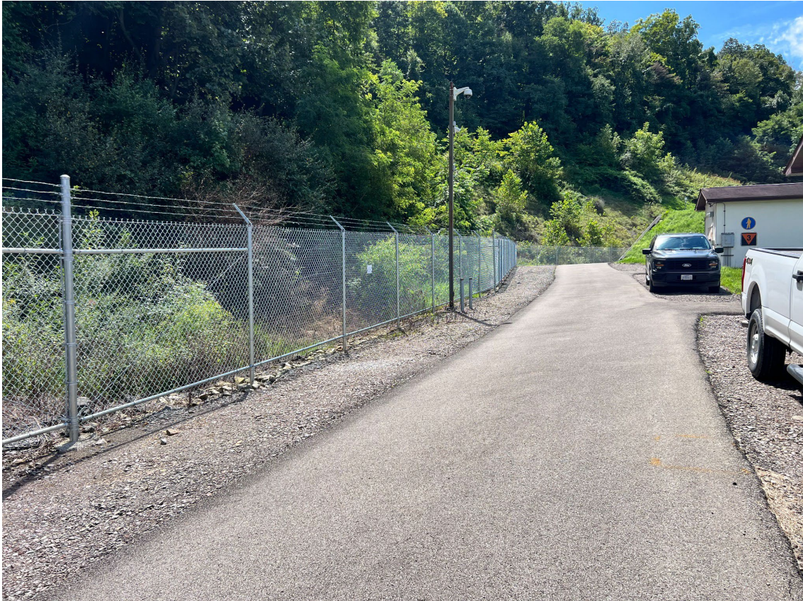
Roadside perimeter section showing good truck access but variable shoulder grade.
