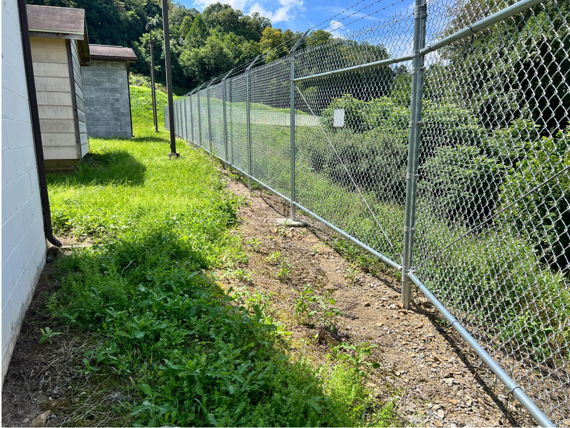
Narrow corridor between the building and fence requiring smaller equipment and phased formwork.
