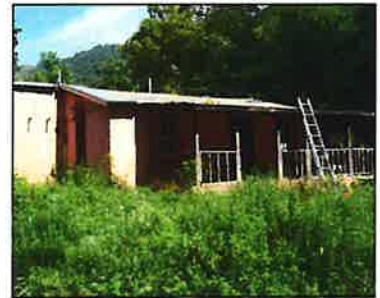
43 structures Logan County, WV
