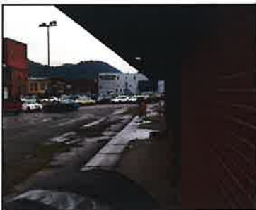
17,600 SF steel frame Kanawha County, WV
