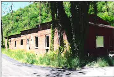
4,000 SF brick structure McDowell, County, WV
