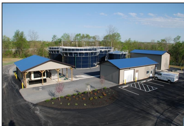
Wastewater Treatment Plant
