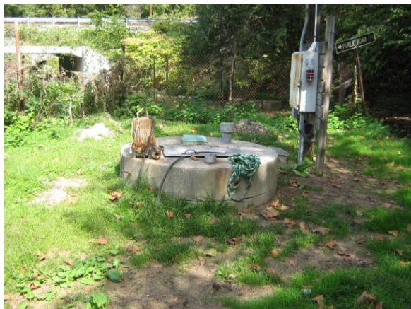
Before: Upper Drive Lift Station
