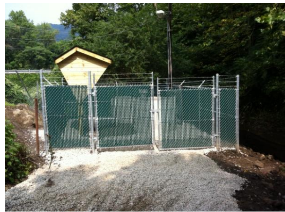
After: Upper Drive Lift Station
