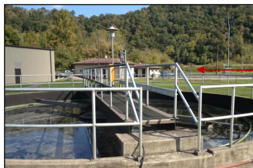
Addition of Third Clarifier
