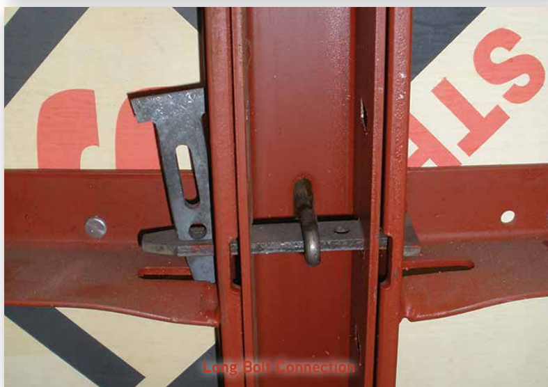
Typical Wedge Bolt Connection
