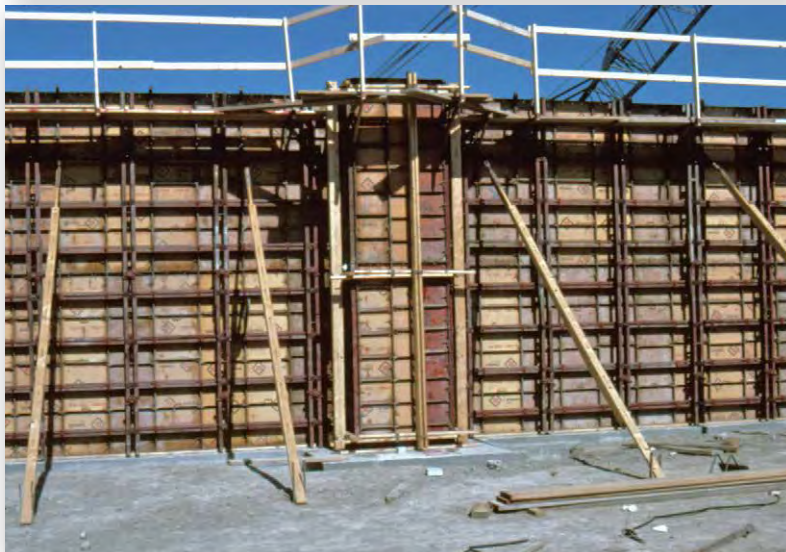
Pilaster Formed with Standard Steel-Ply Components
