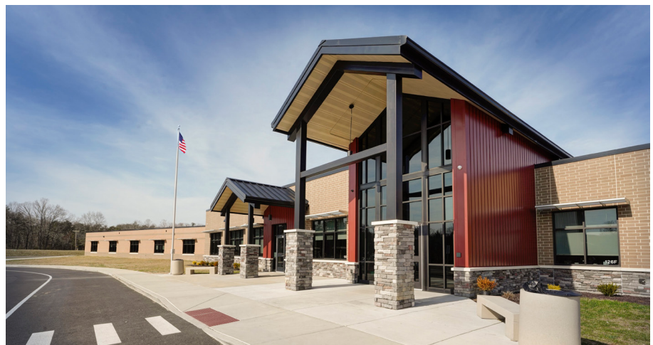
Above: Main entrance of new Peterstown PK8 completed in 2022
