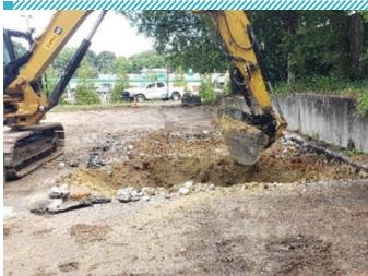
**Atlas was retained by the DSCA Program** for a former dry-cleaning facility utilizing PCE from the 1950s to 2017, when the building was demolished. Concentrations of PCE exceeded soil saturation levels. High Point University purchased the property with the intent of redeveloping the former dry-cleaning site, which would remove the concrete cap overlying the highest area of soil impacts and allow soil to leach into groundwater. Atlas services performed included:
