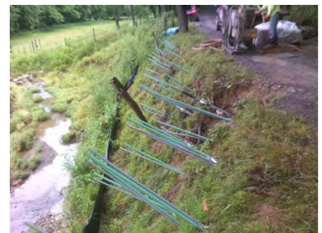
Slide Repair During Construction
