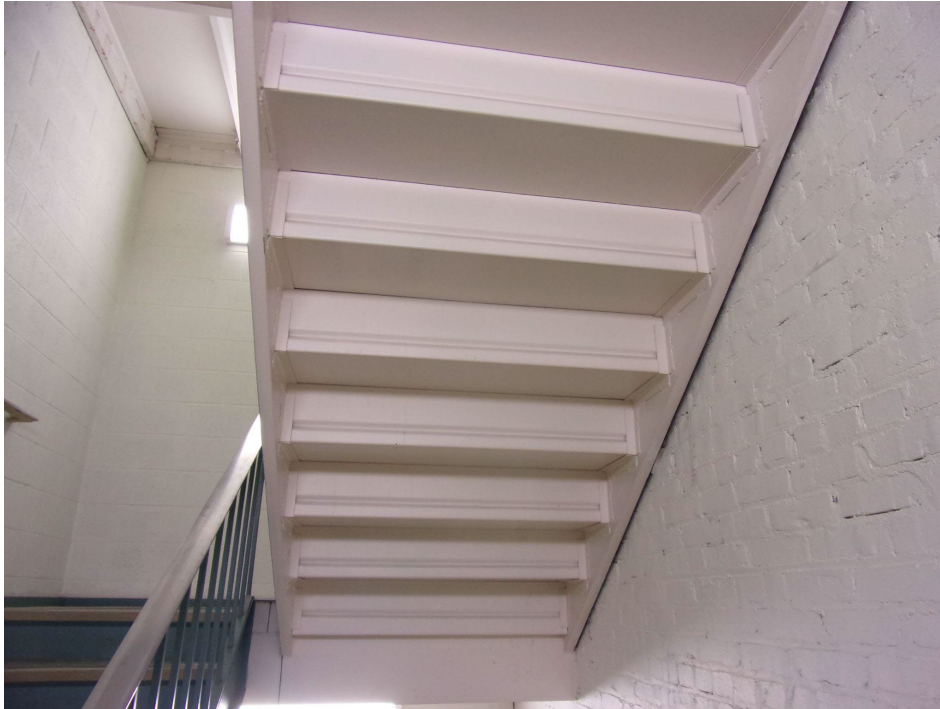
PHOTO 9 North Stair Photo Of Stair Underside
