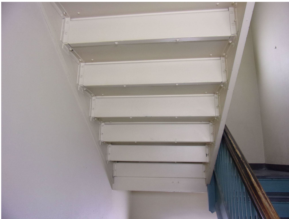
PHOTO 2 South Stair Photo Of The Bottom Side Of The Steps
