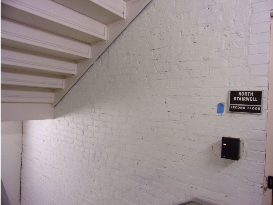
PHOTO 8 North Stair Photo Of Masonry Walls
