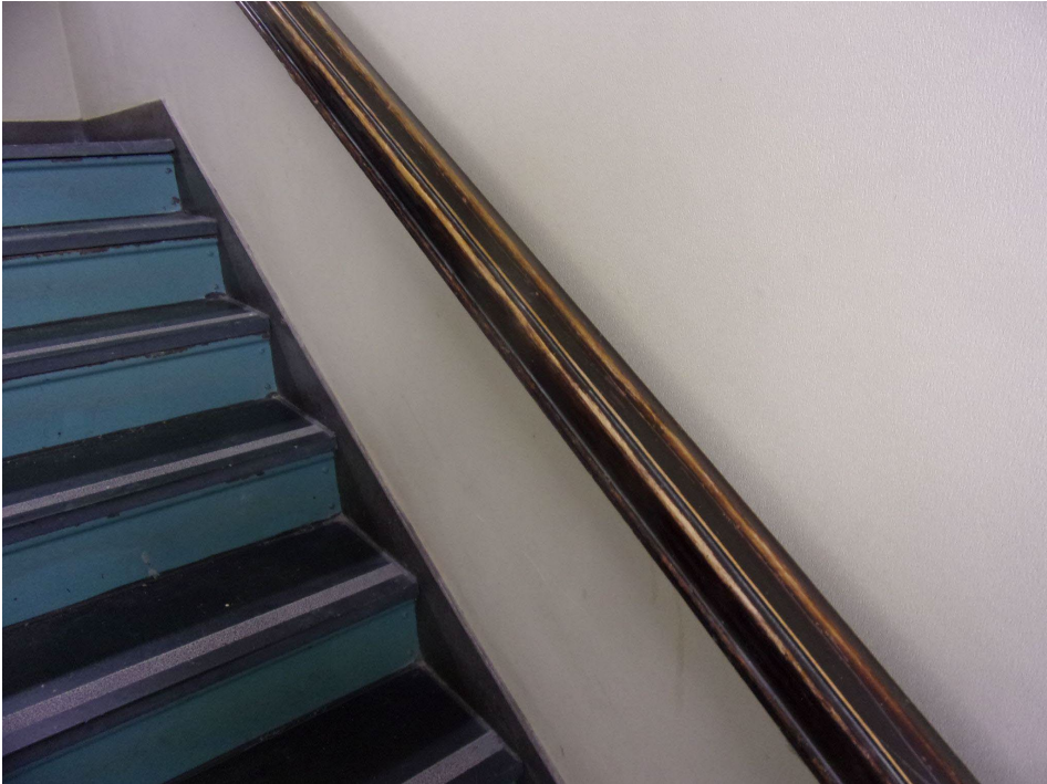
PHOTO 3 South Stair Photo Of Wooden Handrail
