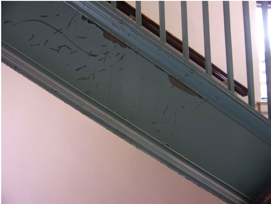
PHOTO 1 South Stair Photo Of The Side Of The Steps
