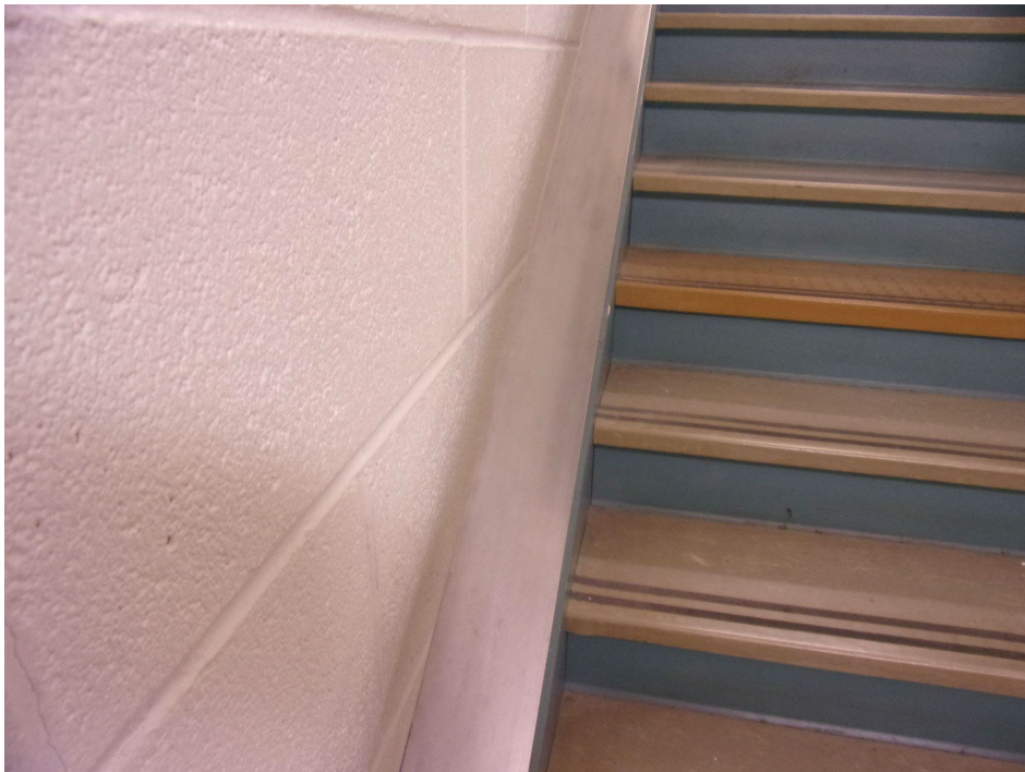
PHOTO 10 North Stair Photo Of Stainless Steel Handrail
