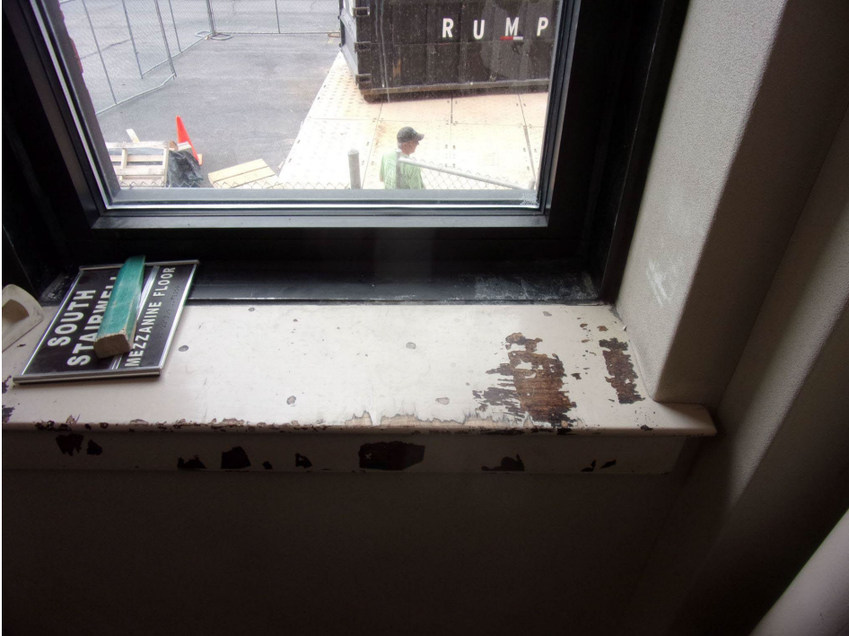
PHOTO 4 South Stair Photo Of Typical Windowsill
