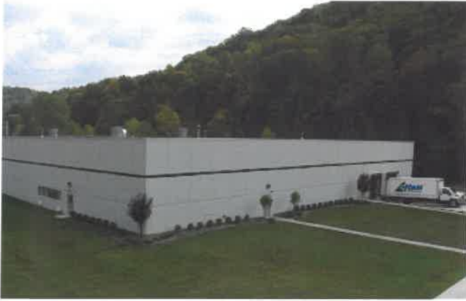
Figure 1: Millennium Center Technology Park
