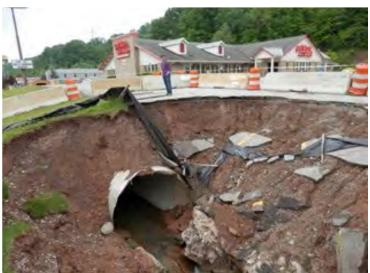
During a storm event in December 2015, a section of 120 inch pipe collapsed in the parking lot of the Golden Corral in Cross Lanes WV. TERRADON was retained by the restaurant owner, Platinum Corral, to determine the best method of repairing the pipe while ensuring the safety of the restaurants customers.
