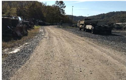
The second road in the project was the ASP Road, a very steep, gravel road that accessed the ammunition bunker. Due to slope and gravel surface, access was often a problem. To accommodate, Alpha designed a specific asphalt paving section which allows forklifts, trucks, and loading equipment to travel with ease.
