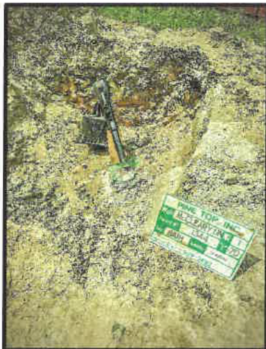
Image 7.2: Post Plug sampling after cutoff
