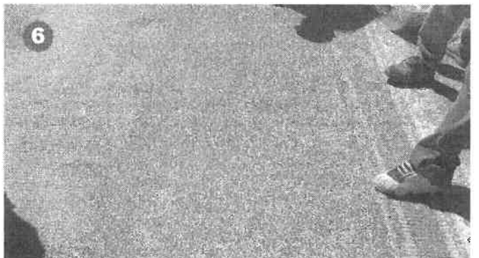
Apply surfacing aggregate to the top layer of TechCrete after it has cooled according to the Installation Instructions.
