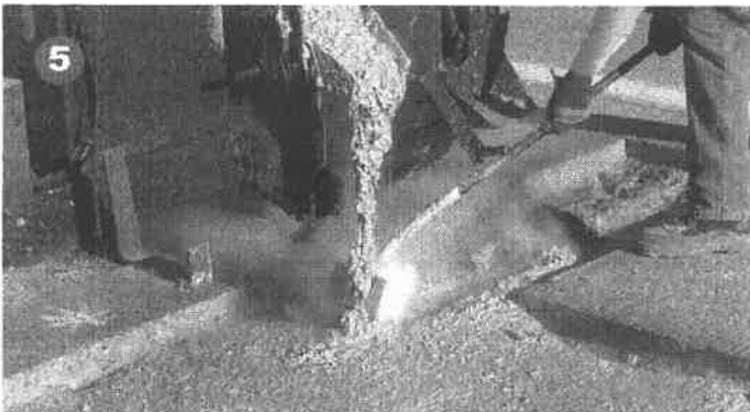
Heat and mix TechCrete in a Crafcro Patcher, as per the directions in the TechCrete Installation Instructions. Pour melted TechCrete into the repair area.
