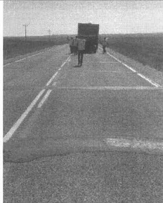
Leveling Depressed Thermal Cracks
