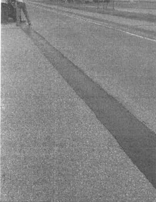
Repairing Deteriorated Longitudinal Joints
