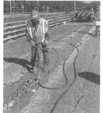
Remove the defective pavement. This may involve saw-cutting, jackhammering, or milling to reach stable pavements.
