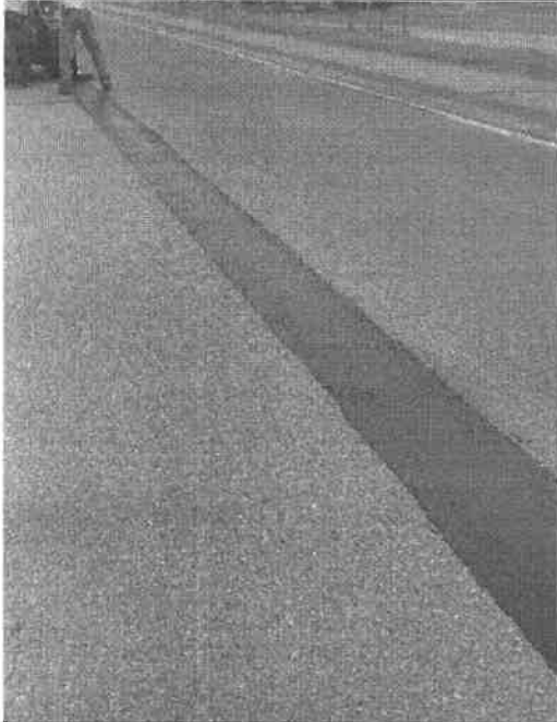
Repairing Deteriorated Longitudinal Joints
