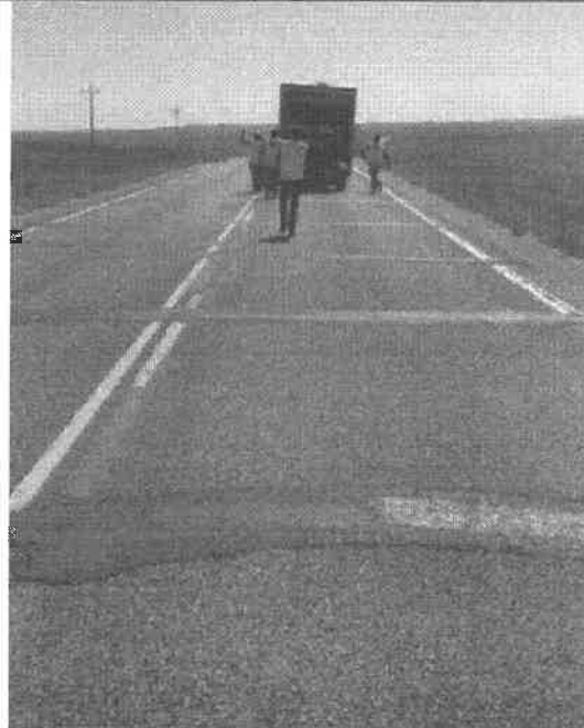
Leveling Depressed Thermal Cracks
