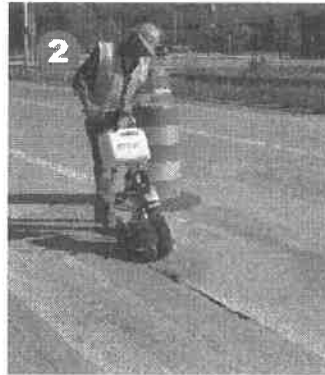
Remove the defective pavement. This may involve saw-cutting, jackhammering, or milling to reach stable pavements.
