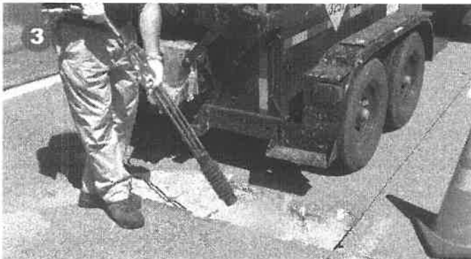
Remove loose debris from the area. Clean and dry the area using a Crafcro Hot Air Lance.
