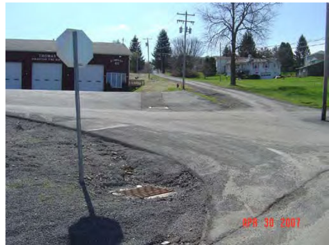
New Storm Drains and Catch Basins
