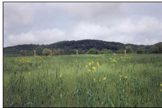
Post construction photograph showing revegetated landfill cap.
