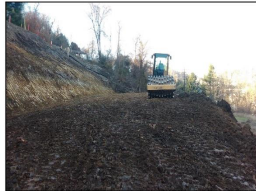
During Construction of Repair
