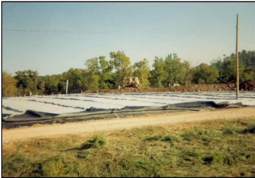
Placement of the final soil cover layer over the geosynthetic layers of the cap.
