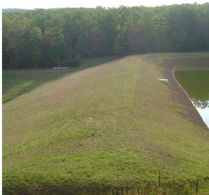
WILSON DAM MODIFICATION, HAMPSHIRE CO., WV
