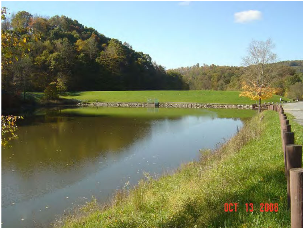
JIMMY LEWIS DAM MODIFICATION, MERCER CO., WV
