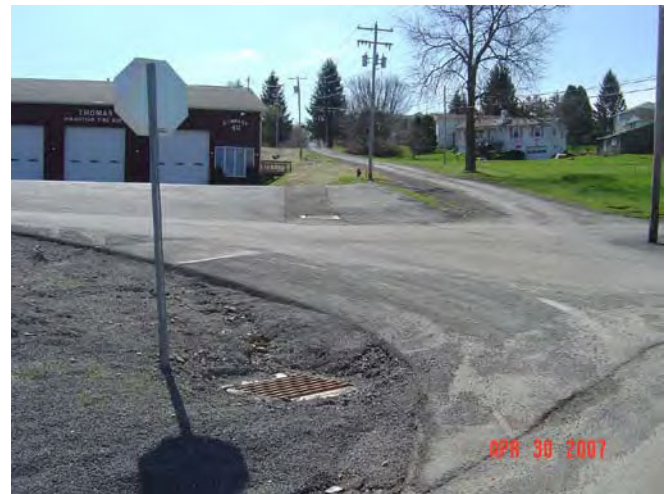
New Storm Drains and Catch Basins
