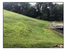
equipping two of the borings with piezometers to measure groundwater levels, and completing a laboratory testing program. Field surveys were completed, and a topographic map developed that served as a baseline map for the design of repair options. A slope stability analysis was performed, and recommendations made for final repair options.
