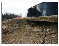
subsurface borings, field testing, and sample collection for laboratory testing. Following completion of the field exploration, POTESTA prepared several regrading alternatives which were analyzed for long-term stability. The final alternative was developed to provide a final slope configuration which included a toe buttress, several rock toe keys/underdrains, and a surface drainage channel to collect, control, and convey surface and groundwater seepage from the regraded fill slope.
