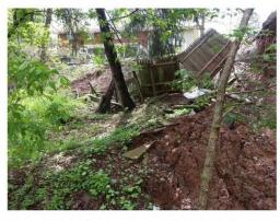
the slope and then working progressively upslope to result in a stabilized and regraded slope surface. The work required the removal of all failed material to the underlying bedrock surface and included the installation of a shot rock toe buttress which was installed along a natural topographic bench near the toe. Following the completion of the slope repair, the affected utilities were installed either below or outside the limits of the regraded slide area.
