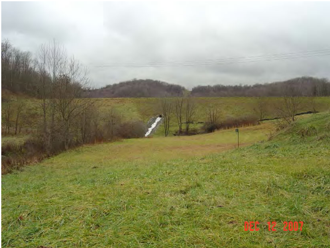
LEMLEY DAM MODIFICATION, MONONGALIA CO., WV
