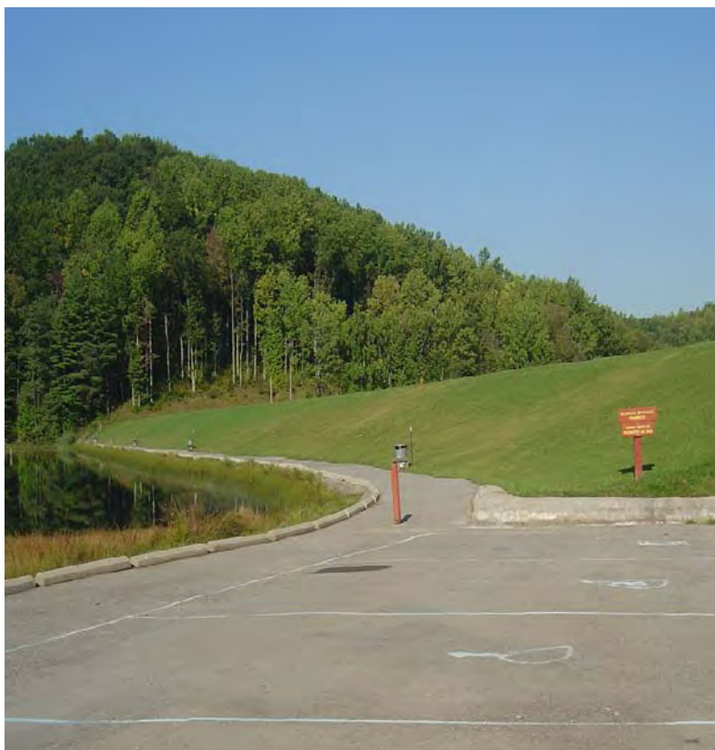
TETER CREEK DAM MODIFICATION, BARBOUR CO., WV
