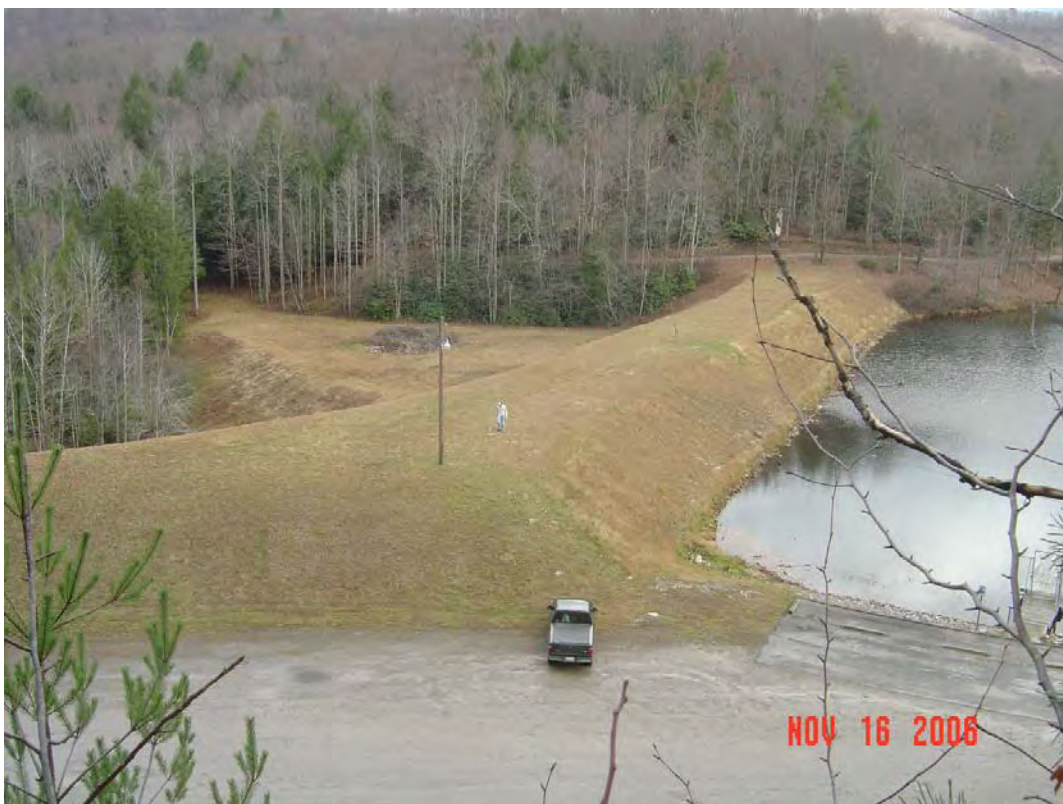
PLUM ORCHARD DAM MODIFICATION, FAYETTE CO., WV
