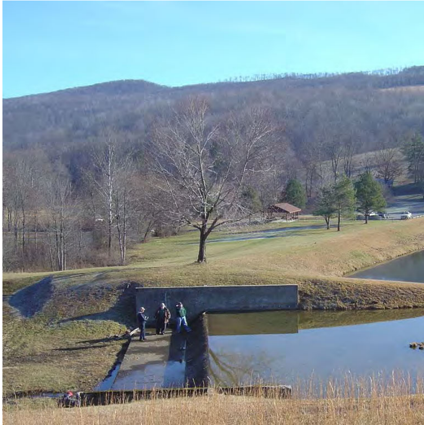
BELINGTON DAM MODIFICATION, BELINGTON, WV
